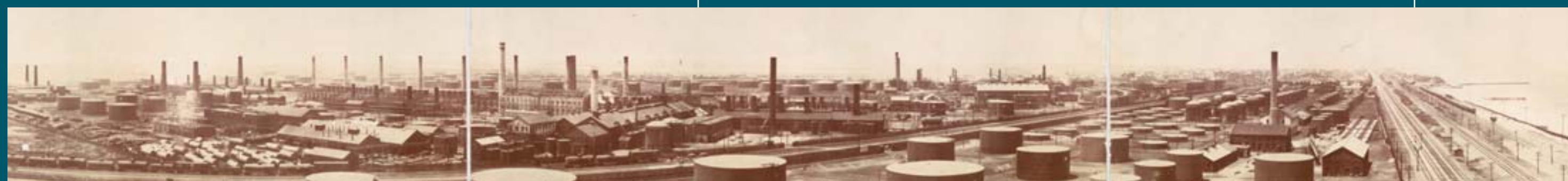
Standard Oil Plant of Whiting, Indiana, by W. H. Wiseman, 1910. LIBRARY OF CONGRESS PRINTS AND PHOTOGRAPHS DIVISION
